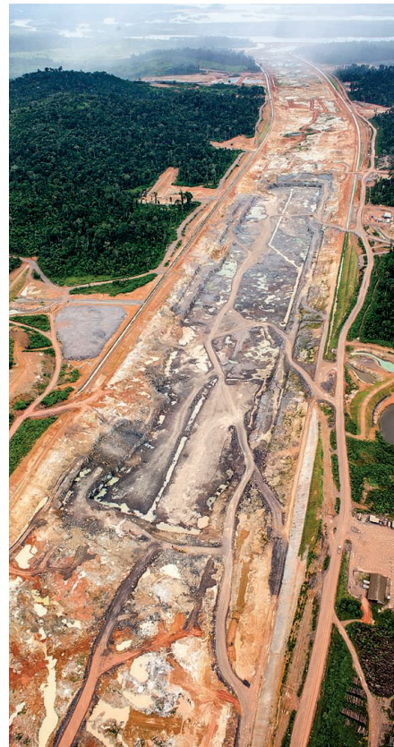
Construction on the Belo Monte dam in Brazil.
